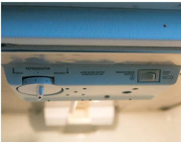
Refrigerator Temperature Controls
