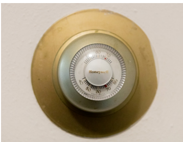
Thermostat (Eagle Heights and Harvey Street)
