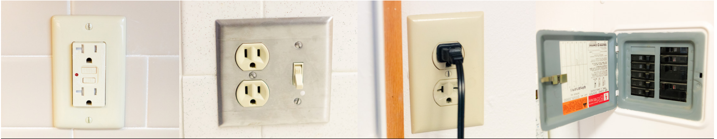
GFCI Outlet (Kitchens and Bathrooms)
