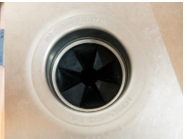
Drain Opening at Bottom of Sink
