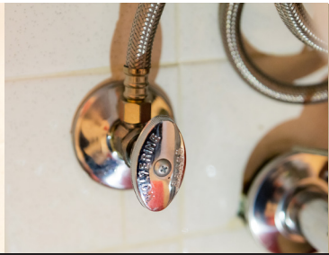
Water Shut Off Valve
