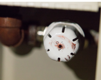
Heat Valve (University Houses)
